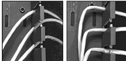
Don't allow the cable to form right angles or sharp bends. Use sweeping bends, no tighter than the curve of a can of Cola.
