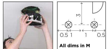
Ensure 1.5m cable coils are left at speaker pre-wire locations to allow for easy installation. Record any pre-wire locations accurately.
