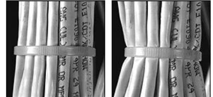
Use tie wraps loosely on large bundles. Do not overstress cables by over tightening cable ties, especially to the point where crush-stress is visible.
