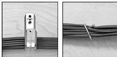
Use j-hooks or similar devices designed to support cables. Do not overstress cables by overloading.
